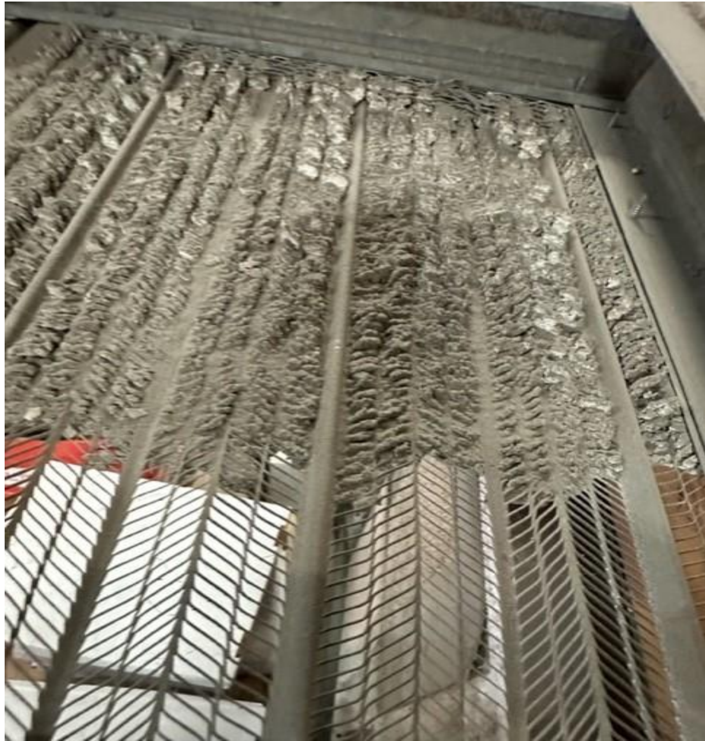
Backside of a Soffit
