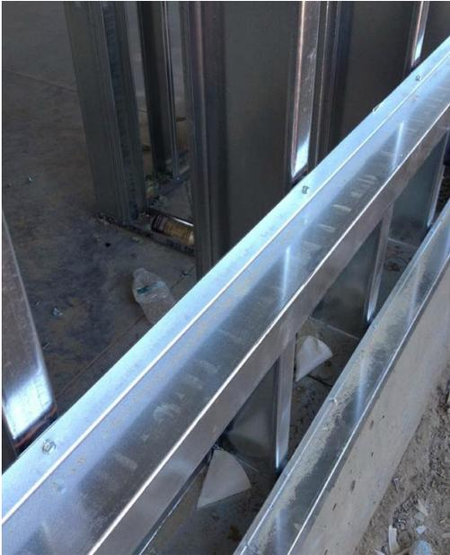
The IECC compliant exterior envelope included a 3 coat plaster assembly utilizing GP Dens Glass Gold sheathing, fluid applied air/water barrier, grade "D" paper and Structa Wire Mega Lath. The assembly successfully "disconnected" the traditional thermal short circuit through the metal studs by horizontally cross furring 16 gauge Z girts and thermally decoupling the connection intersection with plastic "horse-shoe" shims.
