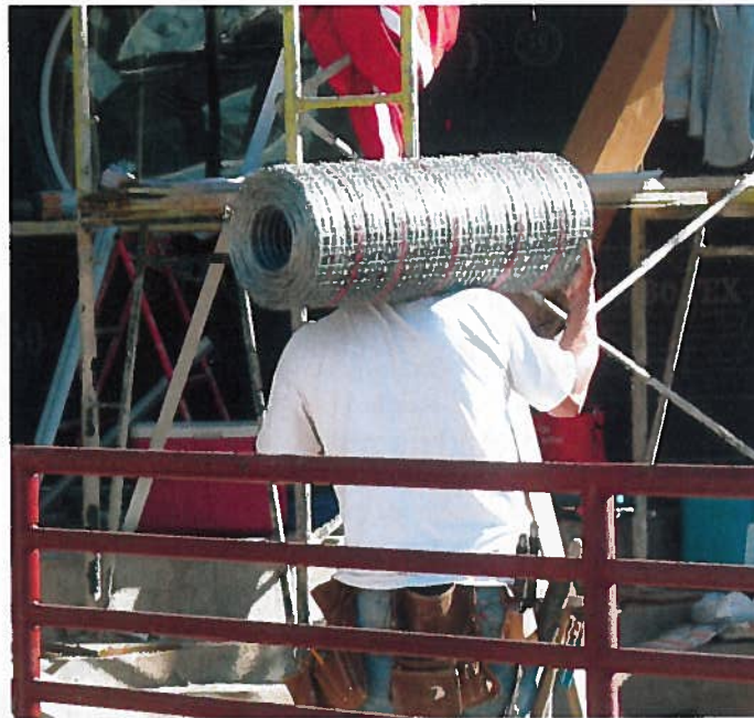
The portability of the self-furred welded wire lath = 25 sheets of sheet lath.
