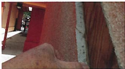
Up close view of self-furred wire embedment in the stucco thickness.
